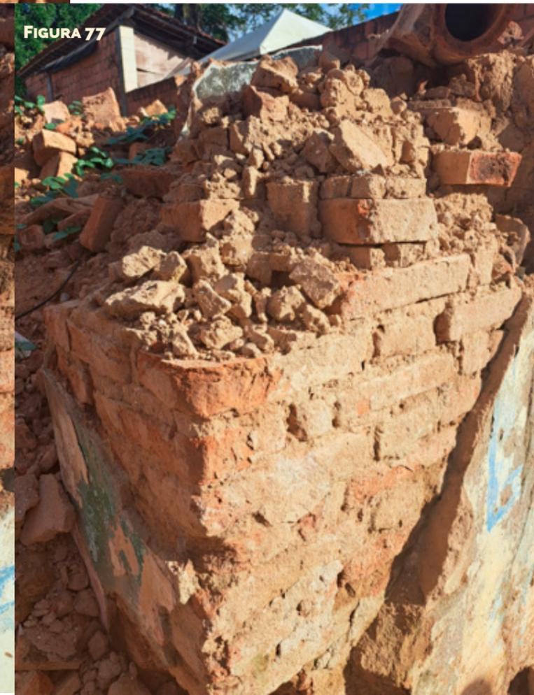
FIGURA 75: DETALHES DA PARTE ESTRUTURAL DOS BLOCOS DE ADOBE FIXADOS NA RESIDÊNCIA ADJACENTE
