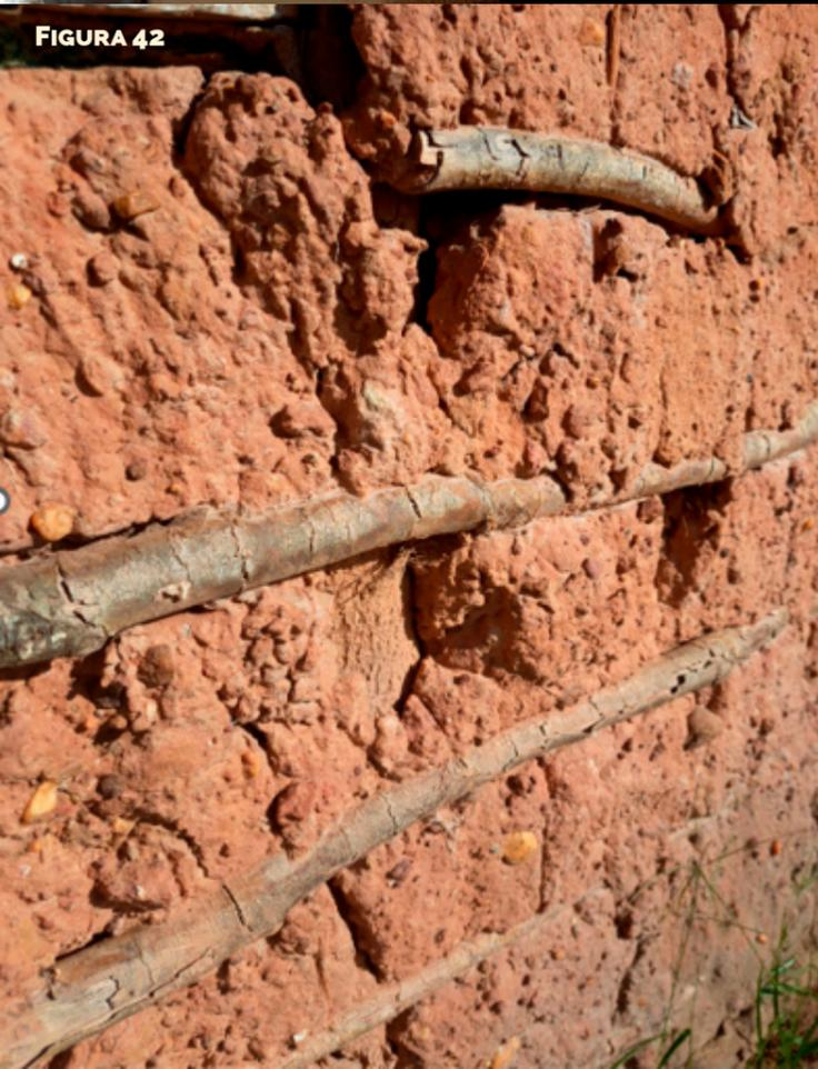
FIGURA 40: DETALHE DA LATERAL, A QUAL ESTÁ APLICADA O REBOCO.
